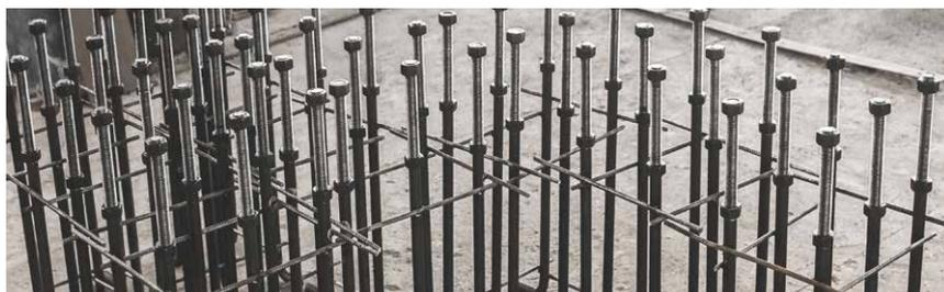
Figure 9: 90° Anchor Bolts Being Set
