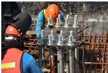
Figure 8: Headed Anchor Bolts Being Set
