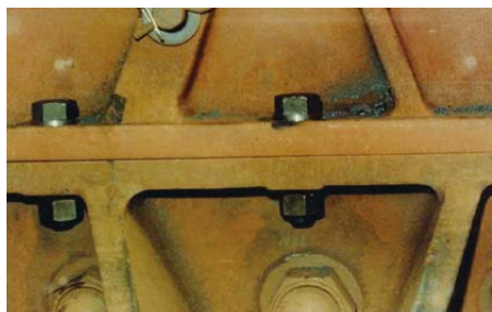
Fig. 8.16 Setup of the CD bolts to side wall
