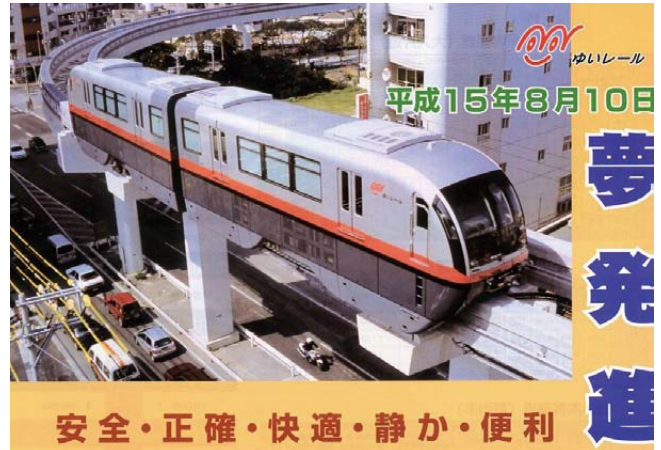
Fig. 8.12 Outer appearance of monorail in Naha City
