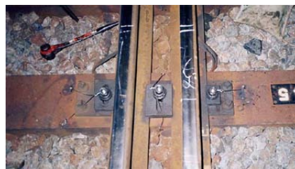
Fig. 8.8 Setup of the CD bolt with strain gauges
