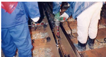
Fig. 8.7 Fastening operation with an impact wrench
