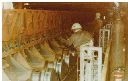
Fig. 8.15 Fastening work of the CD bolt to the side wall of a sintering machine
