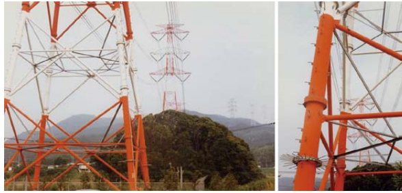
Fig.8.4 Recent steel tower for power supply with pipe
