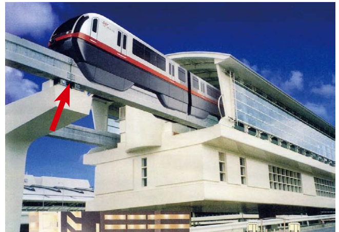
Fig. 8.13 Jointed part of monorail in Naha City
