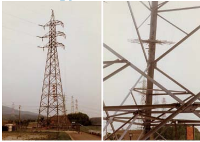
Fig. 8.3 Conventional steel tower for power supply with equal angle
