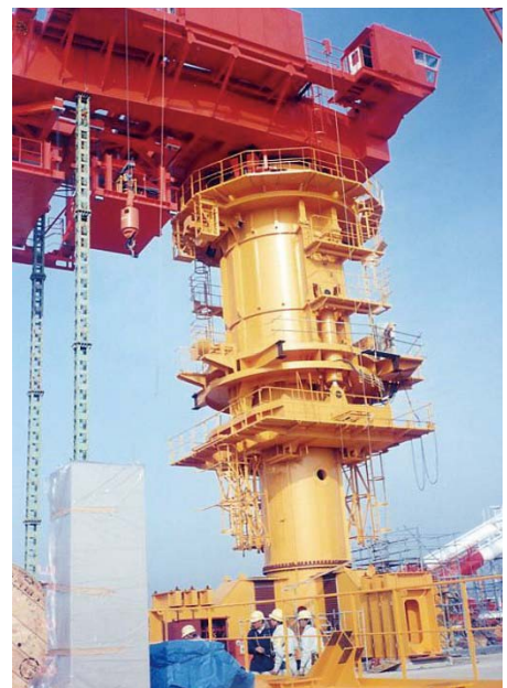
Fig. 8.17 Outer appearance of climbing crane
